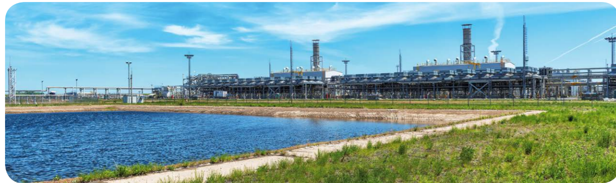
Unit-2 irrigation lagoon
