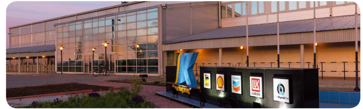
Field Administrative Building at KPC
